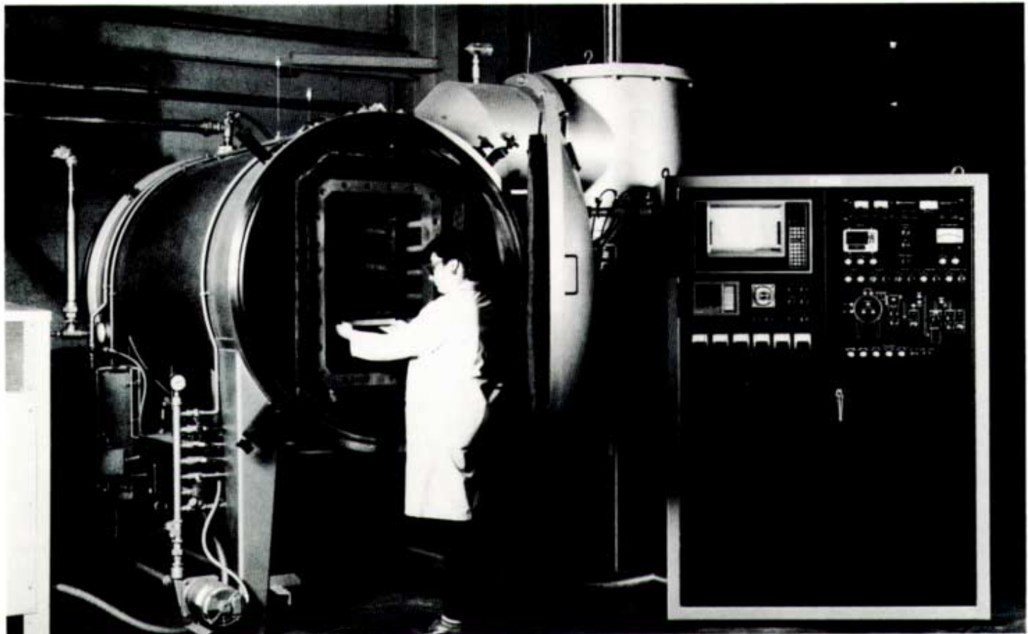
FIG. 5 Injectavac ™ 500 furnace being loaded.
