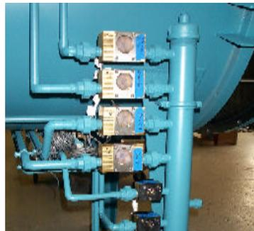
Photograph of closed loop system with Malema flow sensors and integrated flow indicators.
